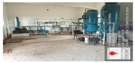
A sewage treatment plant is installed to collect all wastewater generated in the college. It also ensures that the treated water is used for gardening and other activities. The treatment Process/system is designed on the activated Sludge process with Ultrafiltration, which provides the aerobic decomposition of organic matter in the presence of active microbial growthin the aeration tank.
